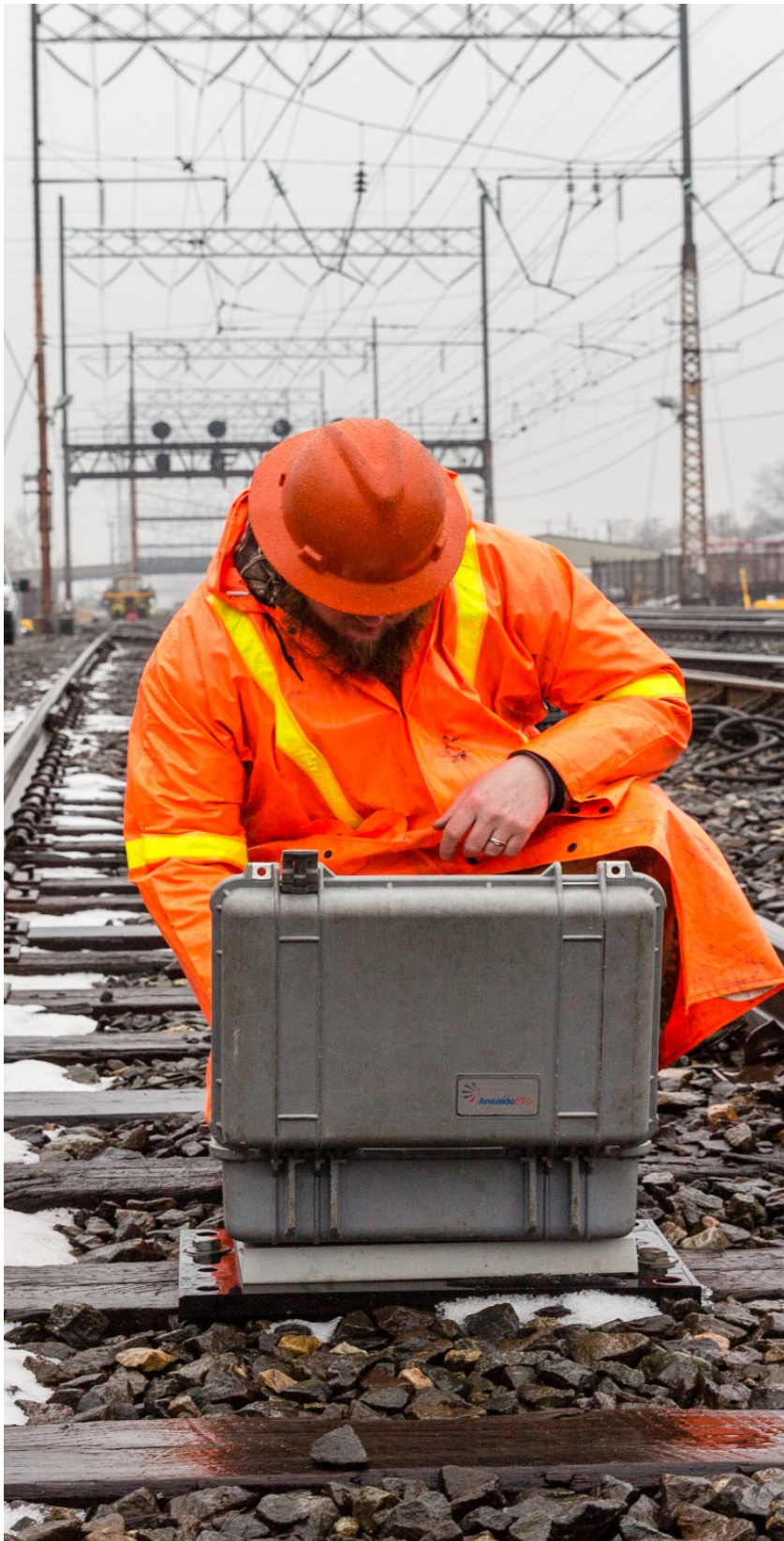
An Amtrak technician resetting a PTC transponder in Pennsylvania along the Northeast Corridor.
