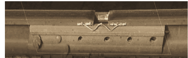
Stripped Joint Bar
