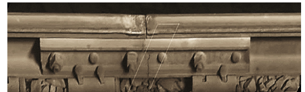
Broken Joint Bar
